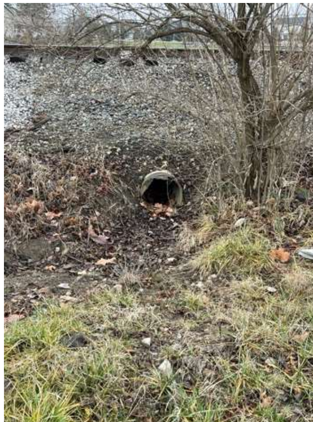
Figure 2-2: 18-Inch Culvert Under Railroad
