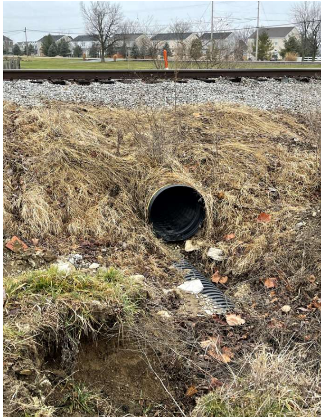
Figure 2-1: 24-Inch Culvert Under Railroad
